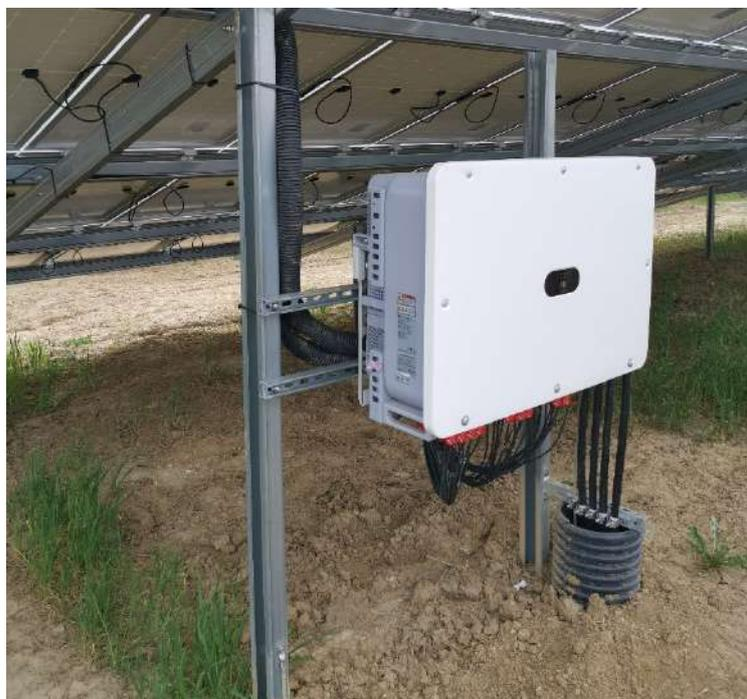
**Figura 3.7 Inverter montato in campo**
